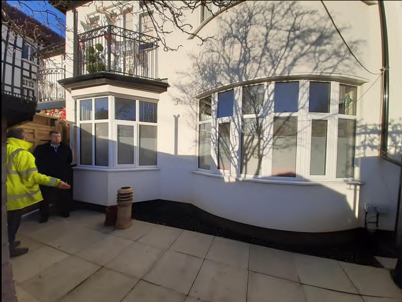
Front part of nursery in enclosed area. Constrc. Manager advised that Early Years department asked for the high fences to prohibit visibility.
